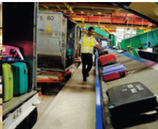
Changi Airport's new Terminal 3 features a high-speed inter-terminal baggage transfer system which can move bags between Terminal 2 to 3 within three minutes.
